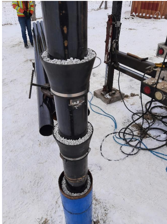
Photograph No. 3 – Bentonite Pellets within Shale Traps – January 18, 2024
