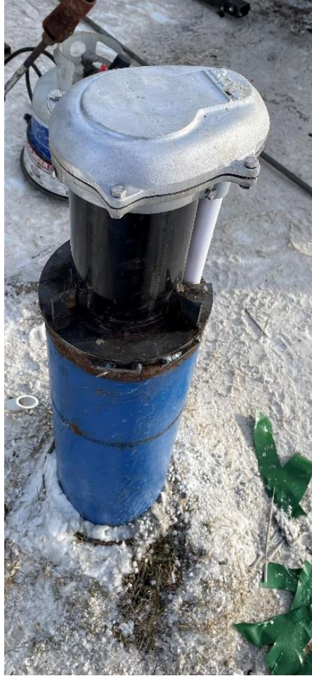
Photograph No. 5 – Completed Installation – January 19, 2024
