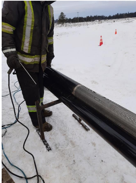
Photograph No. 1 – TW4-24 Stainless Steel Screen – January 18, 2024
