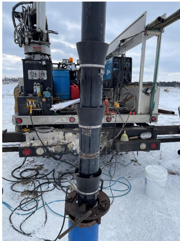
Photograph No. 2 – Installation of Shale Traps – January 18, 2024
